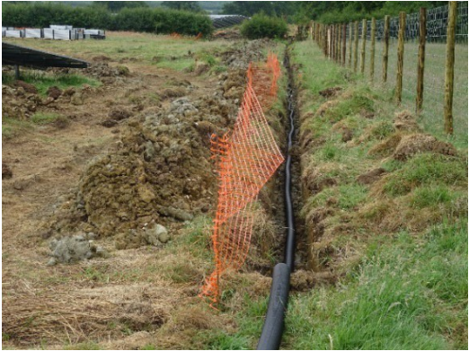
Inserts 38 and 39: Cable Installation
