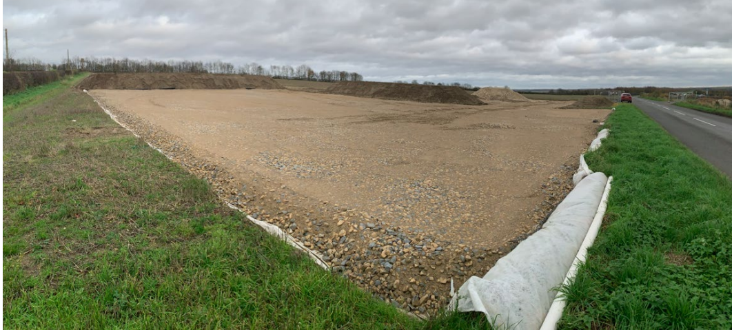
Insert 2: Example temporary construction compounds
