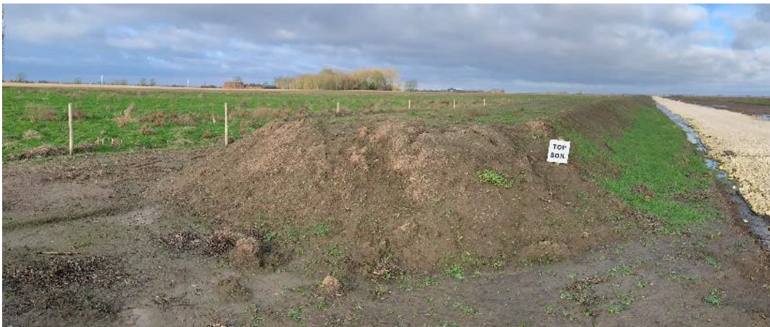
Insert 8: Temporary Topsoil Storage (January 2023)
