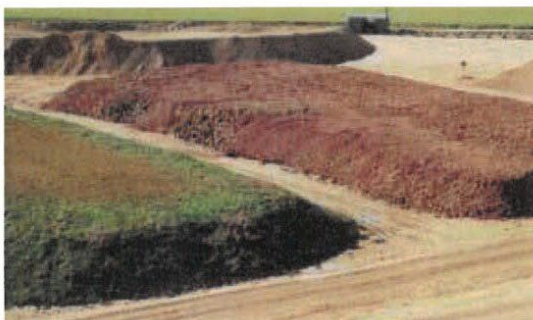
Clearly defined stockpiling of different soil materials
