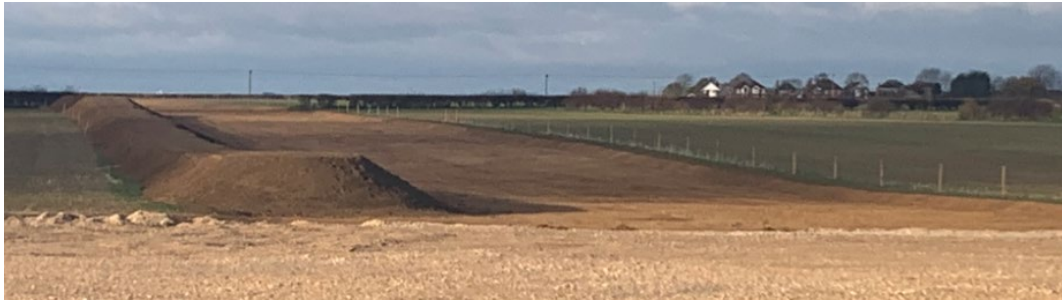
Insert 3: Example stripping of topsoil across the working width
