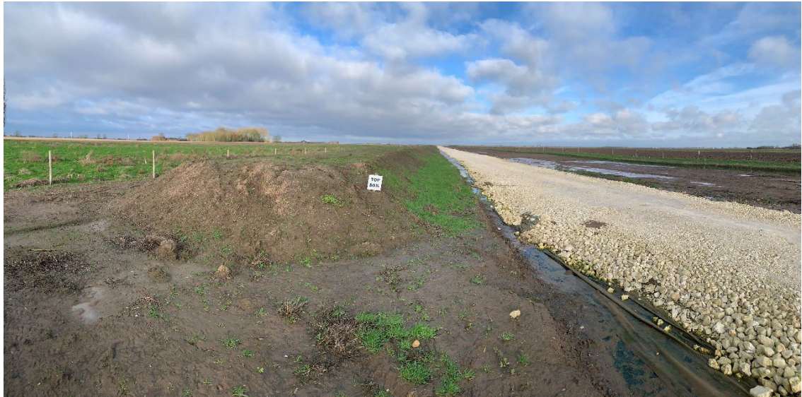
Insert 13: Temporary Topsoil Storage (January 2023)
